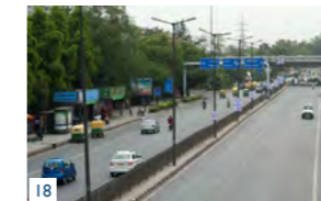
18 Signage, guardrails, lighting etc. facilitating the carriageway
