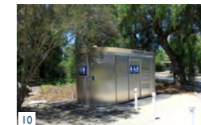
10 Facilities on the MUZ along the pedestrian walkway
