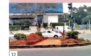
32 Absence of kerb ramps
