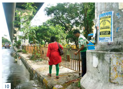
10 Discontiguous guardrails allowing people to detour onto the carriageway
