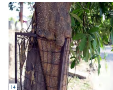
14 Tree guards not accommodating the tree girth.
