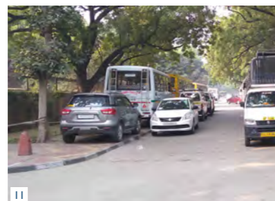
11 Kerb height less than 150mm allow vehicles to encroach onto the walkway
