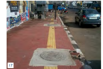
17 Tactile paving obstructed my manholes cover
