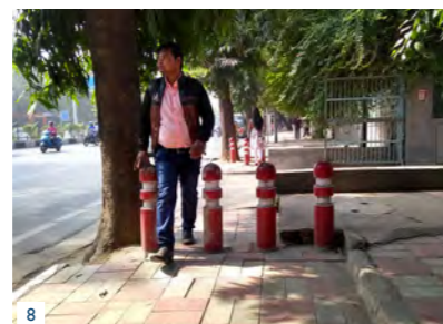
8 Bollards placed with no provision for wheelchair users
