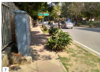
7 Feeder Pillar obstructing walkway
