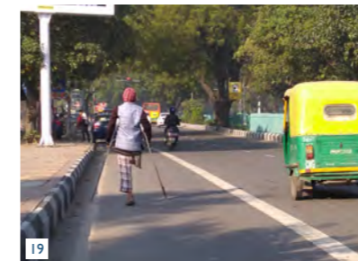
19 Absence of Kerb ramps
