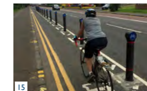
15 Reflective bollards segregate the NMV on the carriageway
